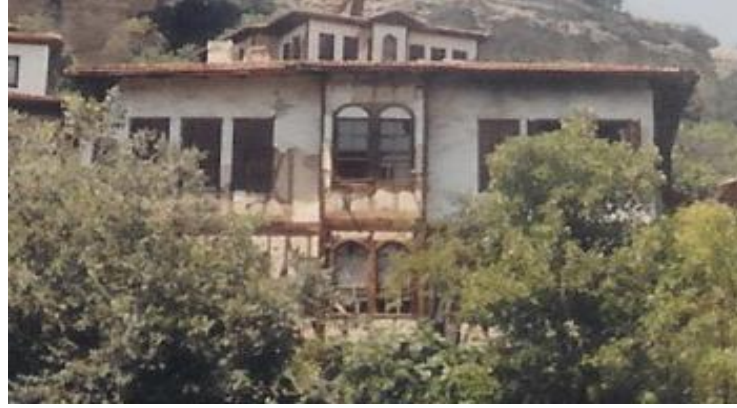
Figure 2. Front view of the building numbered 1.
