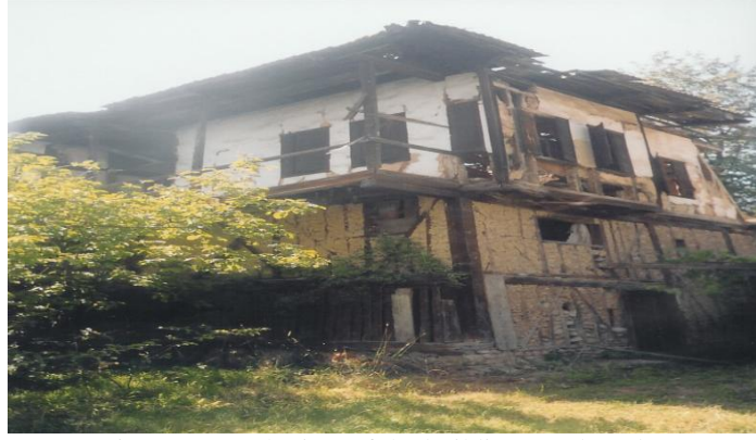
Figure 5. North view of the building numbered 4.
