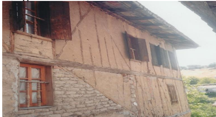
Figure 3. Side view of the house numbered 2.
