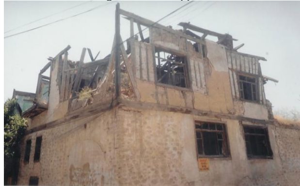
Figure 9. Side view of the house numbered 8.
