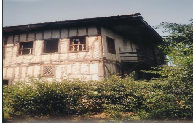
Figure 8. Side view of the house numbered 7.
