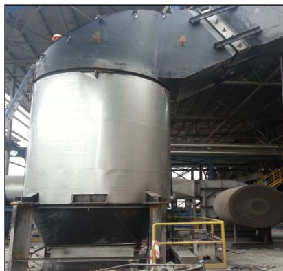
Figure 2. Economiser assembly picture.
